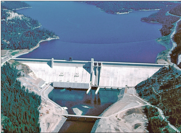
Libby Dam, Montana
