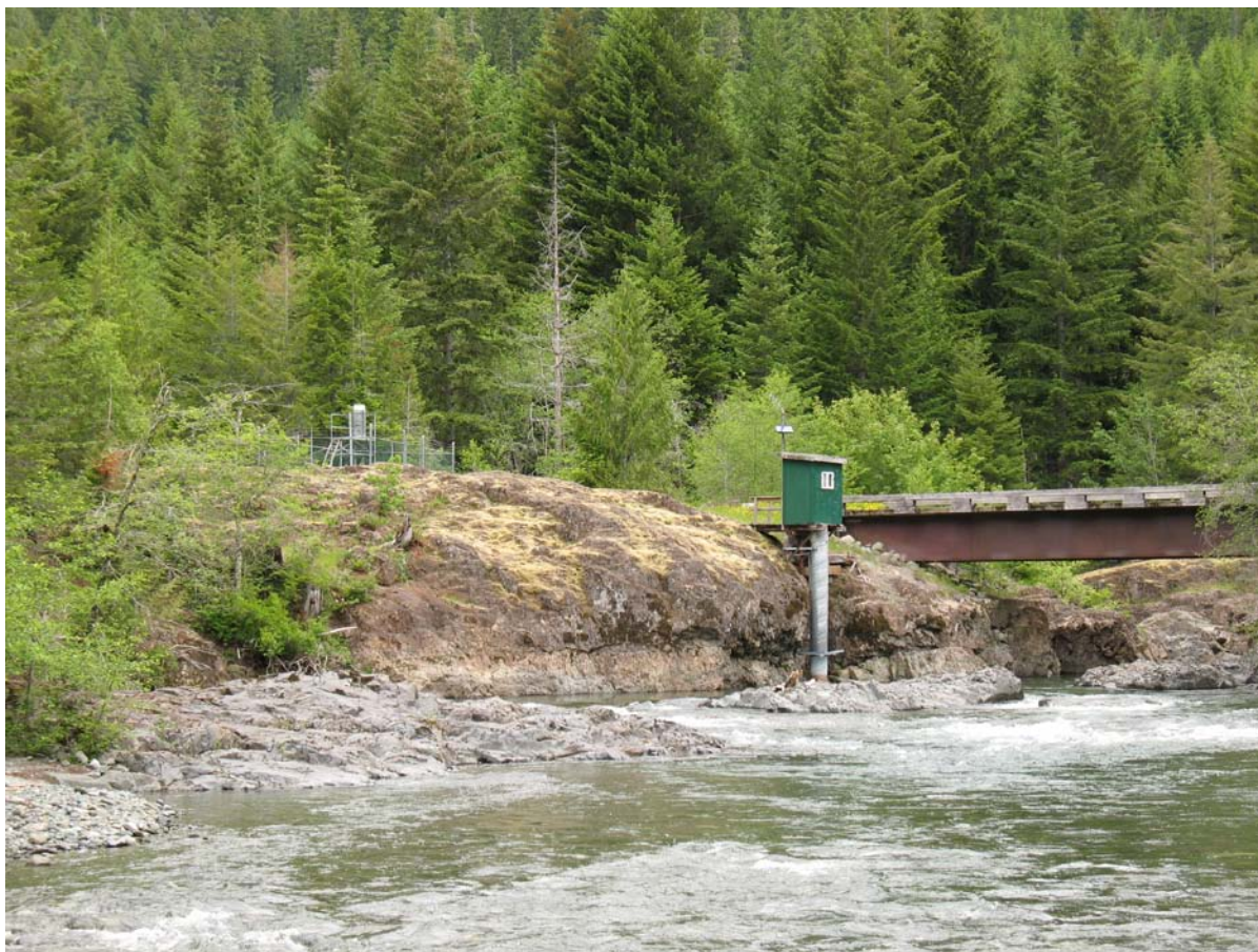
Climate and River Level Monitoring Station, Elk River (BCH)
