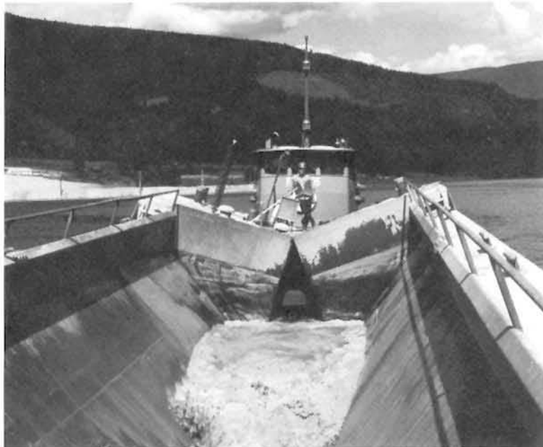
BOTTOM DUMPING BARGE used in construction of Hugh Keenleyside Dam
