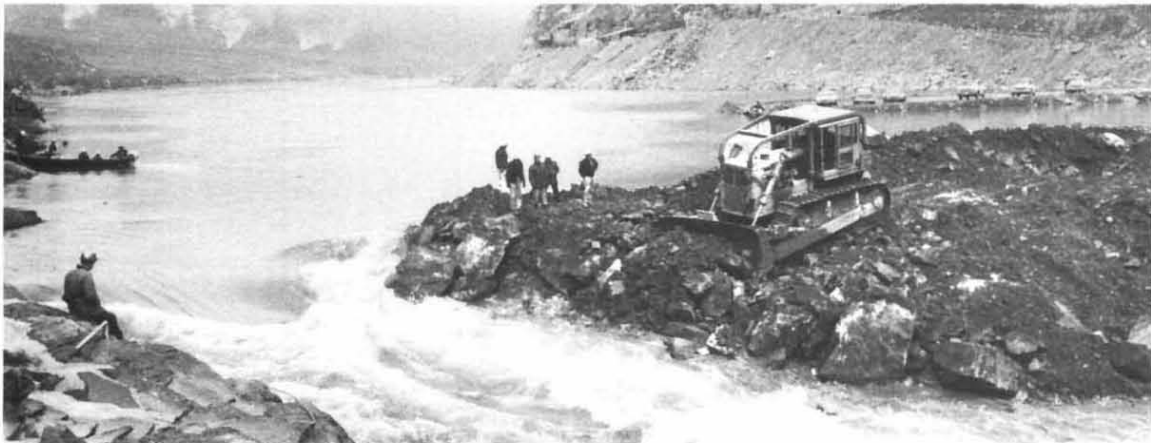
CLOSING COFFERDAM at Mica Dam in 1967
