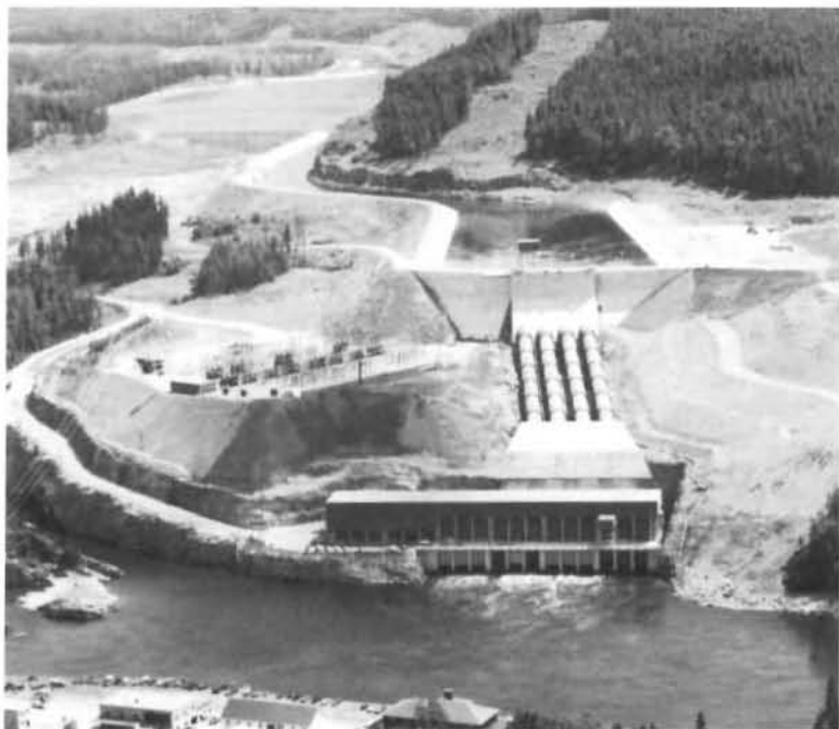
KOOTENAY CANAL PLANT made possible by Treaty storage
