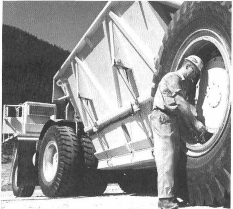
EARTH-MOVING MACHINERY at Mica Dam, 1969.
