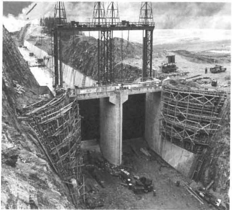
SPILLWAY CONSTRUCTION at Duncan Dam in 1967.
