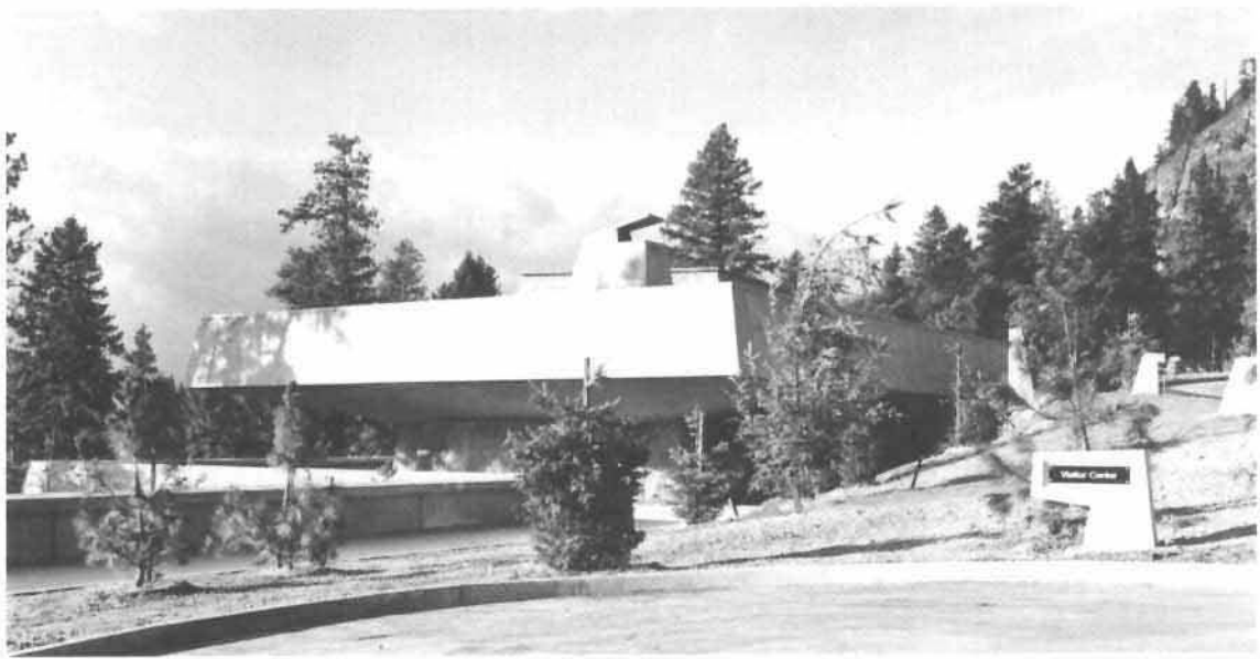
VISITOR'S CENTRE at Libby Dam.
