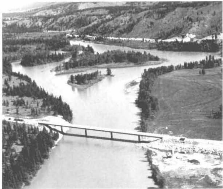
WARDNER BRIDGE nearing completion in 1972, Lake Kookanusa in British Columbia.
