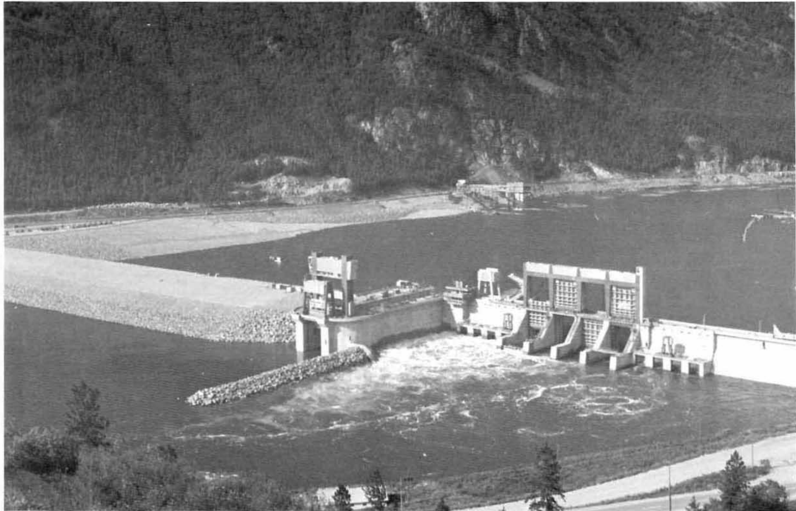
HUGH KEENLEYSIDE DAM Concrete spillway and discharge works with navigation lock and earth dam.
