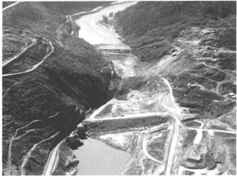
MICA DAM CONSTRUCTION during 1967, looking downstream.
