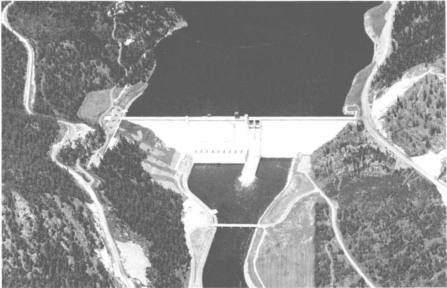
LIBBY DAM The dam and reservoir, Lake Koocanusa. The powerhouse is at the left of the spillway. Kootenai River, Montana
