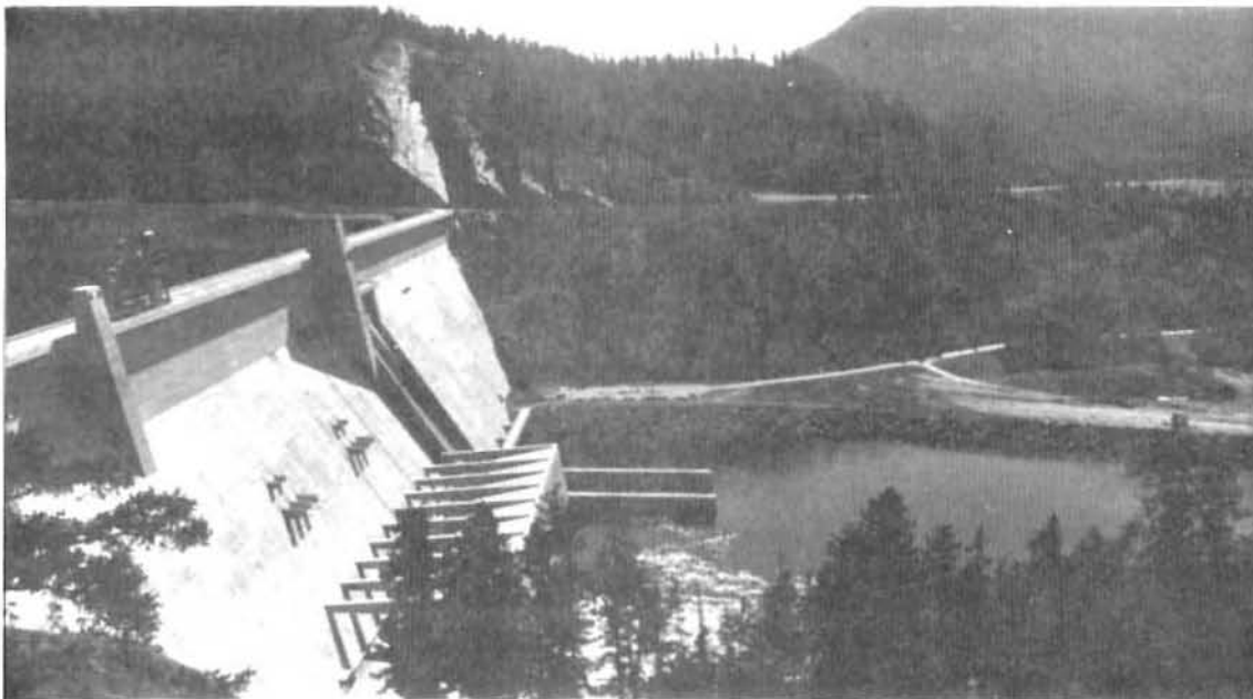
LIBBY DAM and POWERHOUSE on Kootenai River in Montana.
