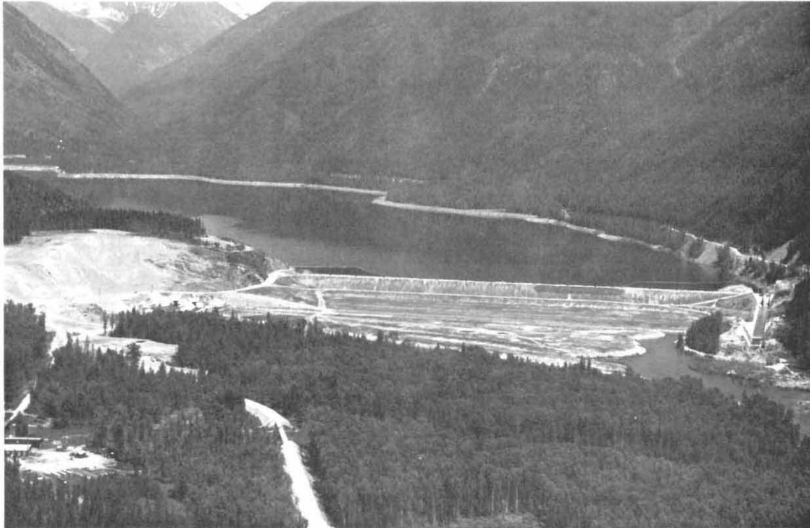
DUNCAN DAM The earth dam with discharge tunnels to the left and spillway to the right.
