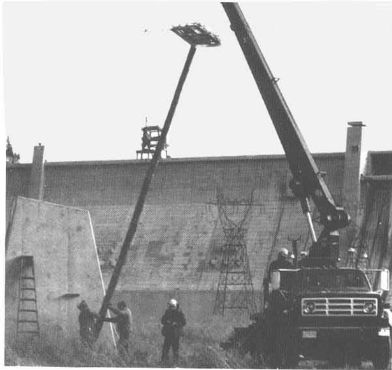
INSTALLING NESTING PLATFORMS at Libby Dam, Montana.
