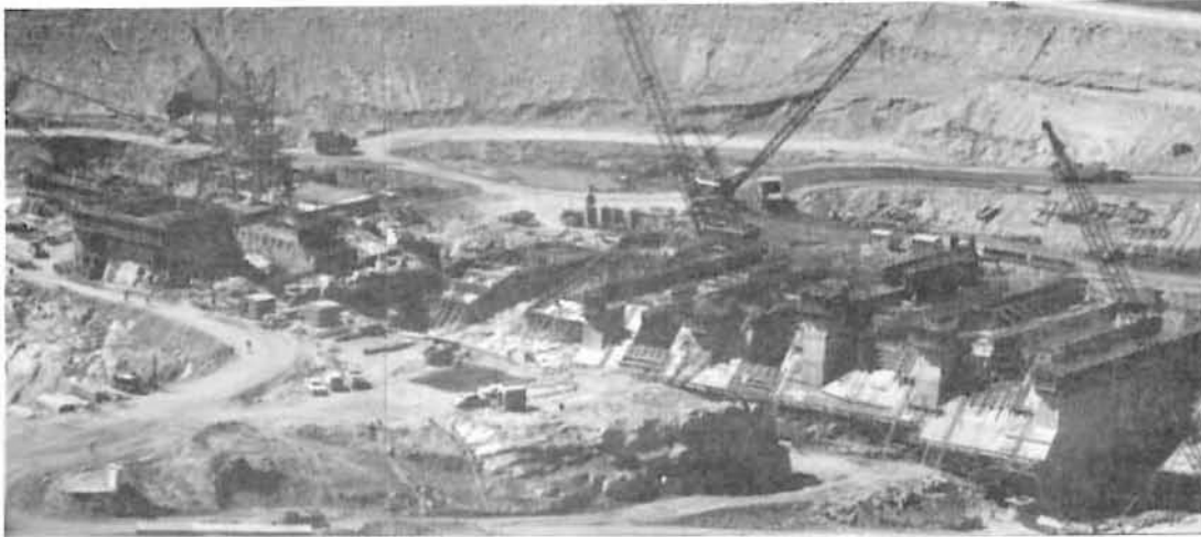
SPILLWAY and LOCK CONSTRUCTION, Hugh Keenleyside Dam in 1966.
