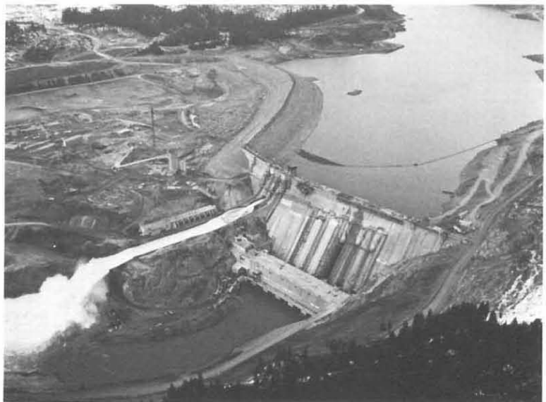
REVELSTOKE DAM downstream from Mica Dam completed in 1984.
