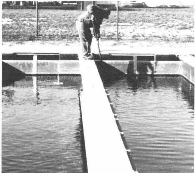
FISH HATCHERY at Murray Springs, Montana completed October 1979.
