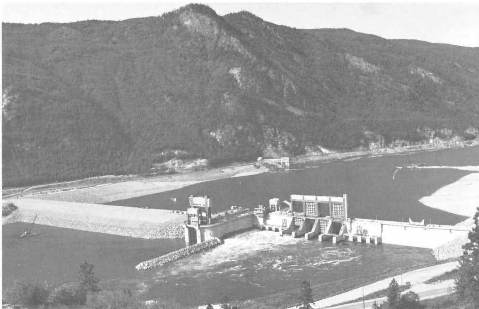
HUGH KEENLEYSIDE DAM Earth dam at the outlet of Arrow Lakes with navigation lock and discharge works.
