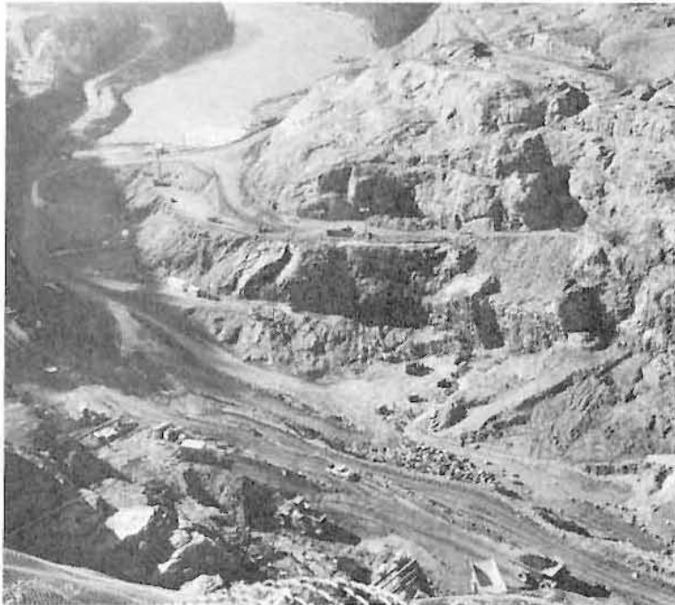
REVELSTOKE PROJECT downstream cofferdam and excavation for concrete dam and powerhouse.
