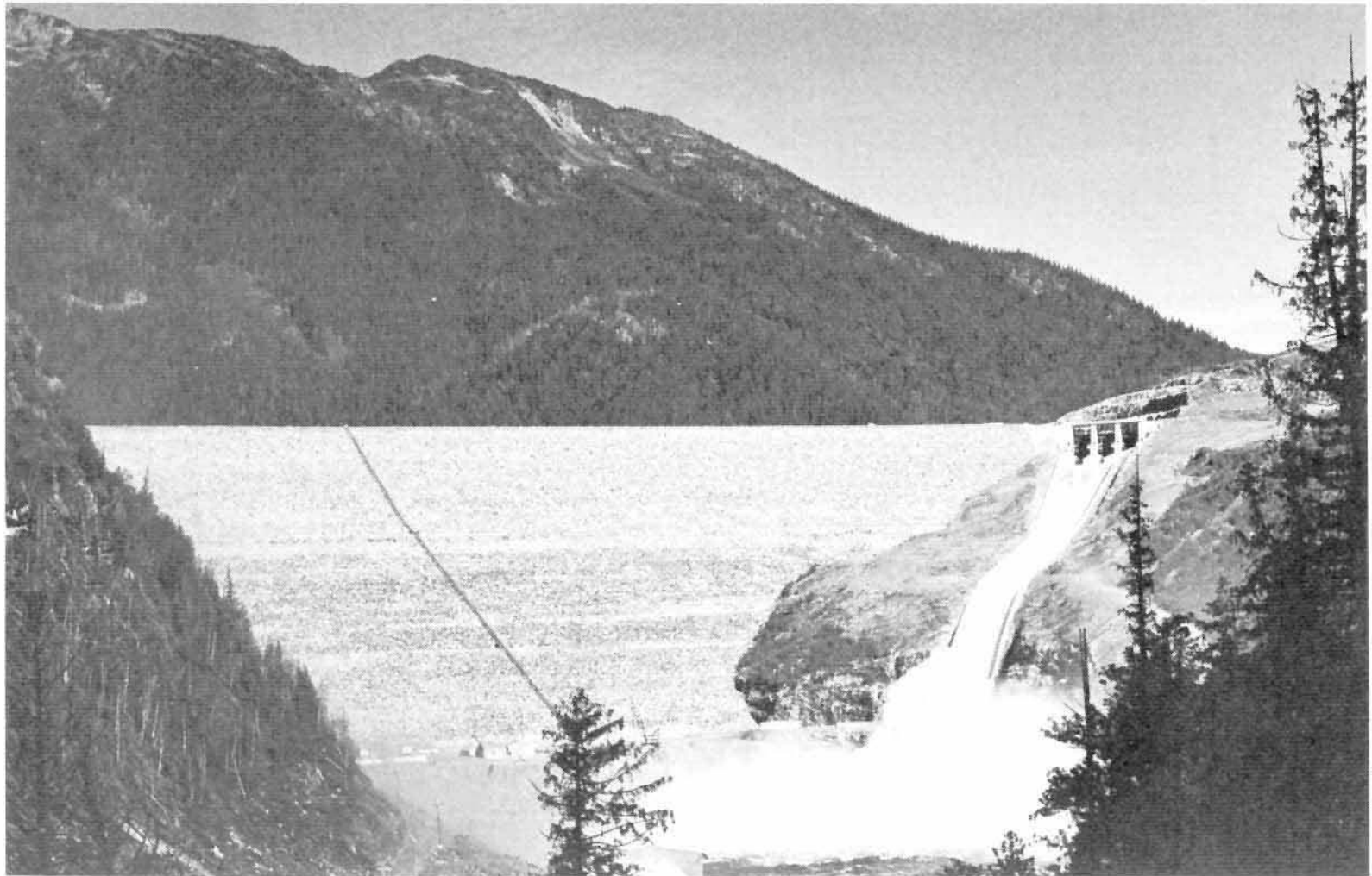
MICA DAM The earth dam with the spillway in use.
