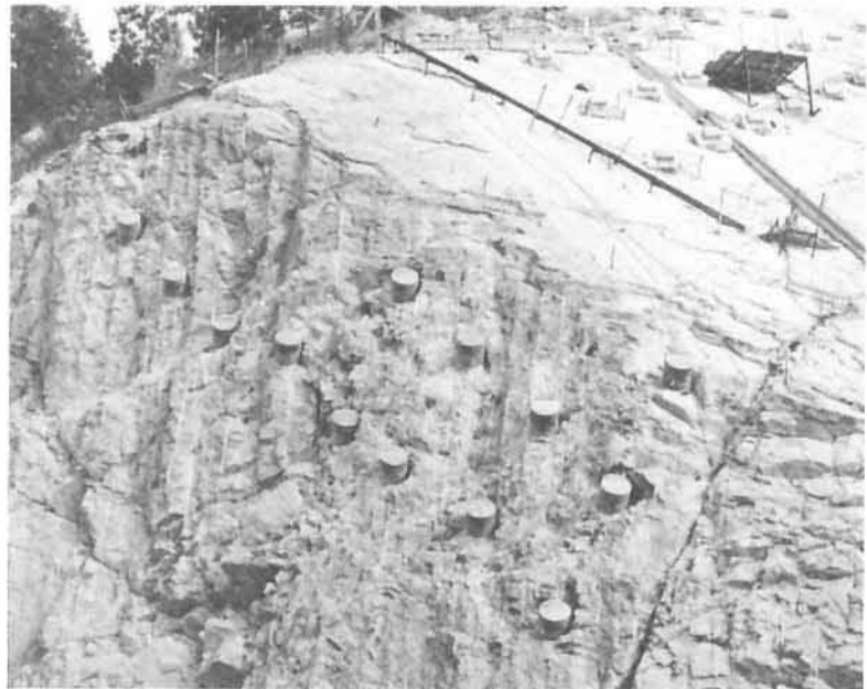
ROCK STABILIZING capped steel tendons eliminate slide danger at left abutment of Libby Dam.
