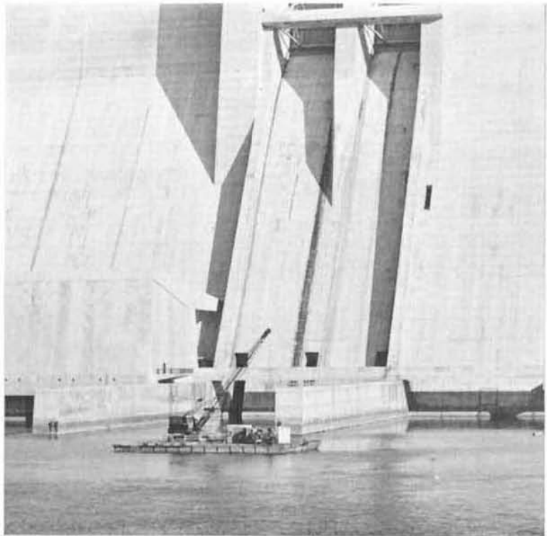
STILLING BASIN for spillway at Libby Dam undergoing concrete repairs.
