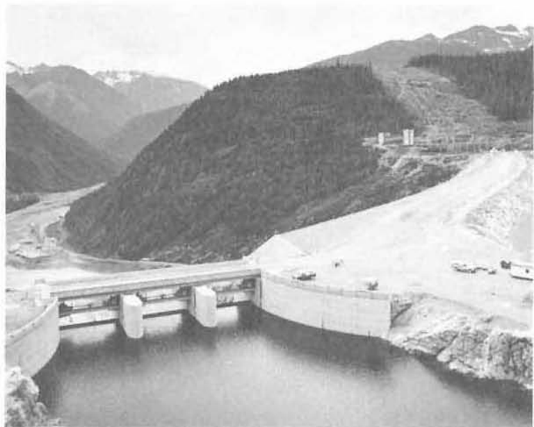
SPILLWAY CONTROL structure and crest of Mica Dam.
