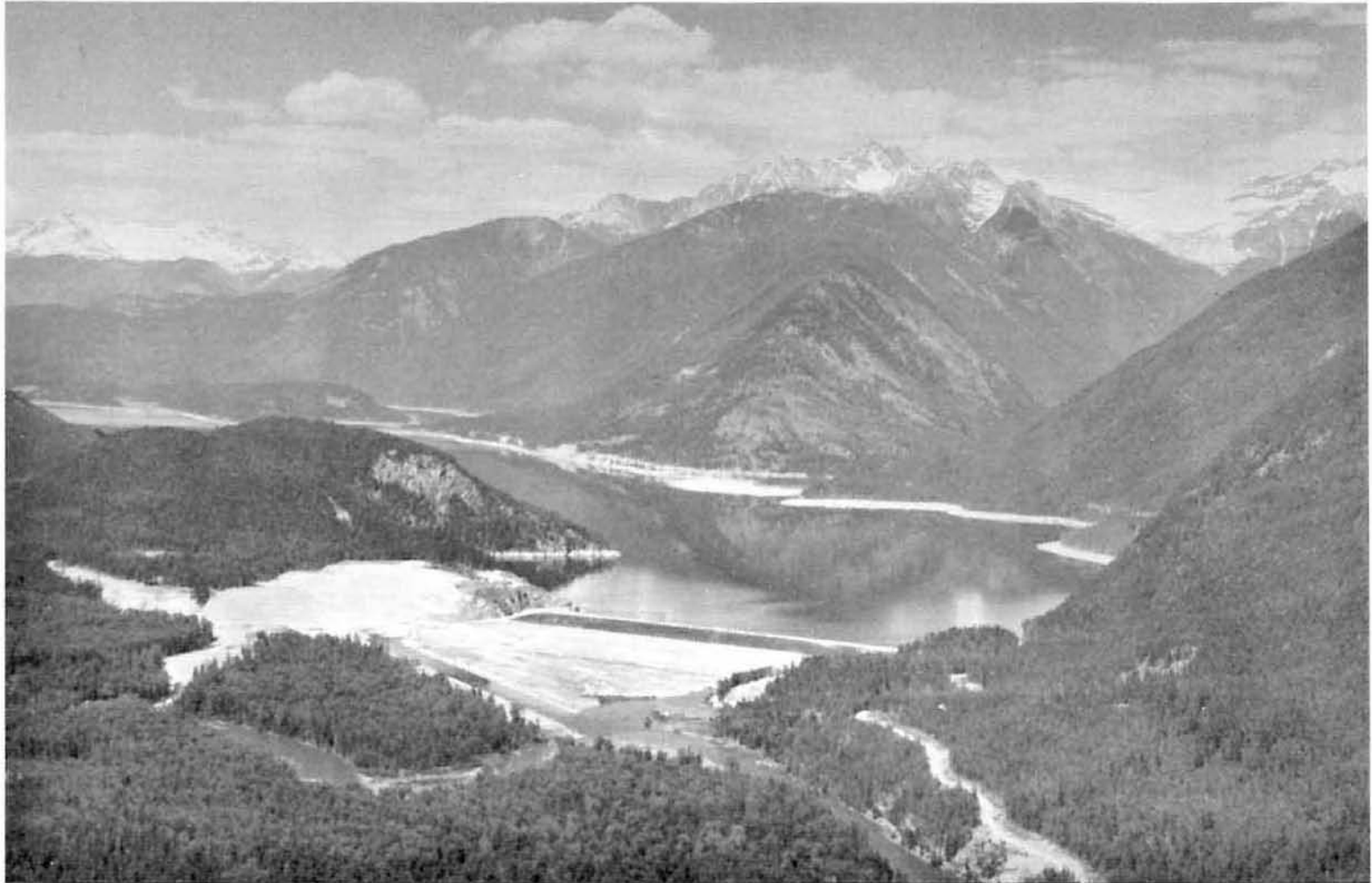
DUNCAN DAM The dam and Duncan Lake.
