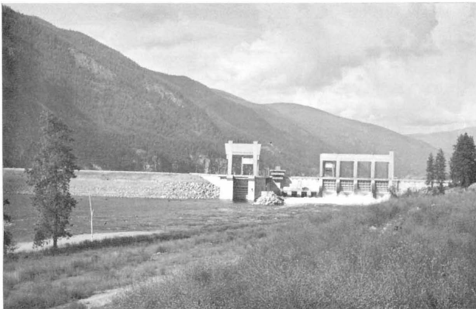
HUGH KEENLEYSIDE DAM
