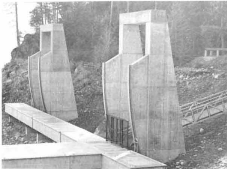
SMALL BOAT MOORAGE at Souse Gulch on Lake Kooconusa designed to move with changing reservoir level.
