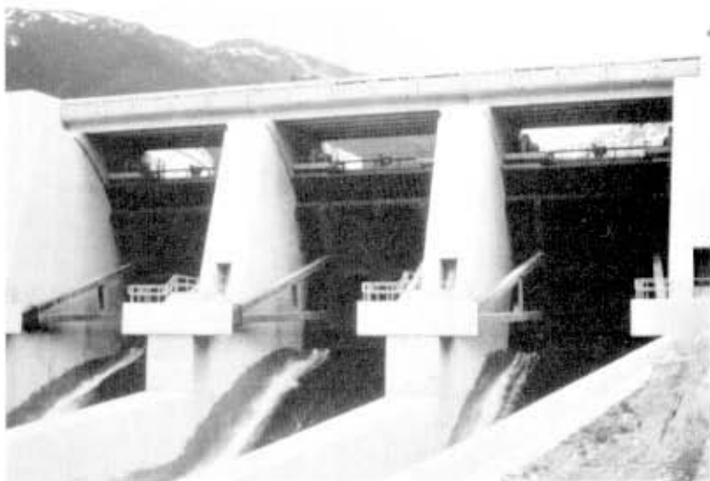
SPILLWAY GATES in use at Mica Dam, July 1976.
