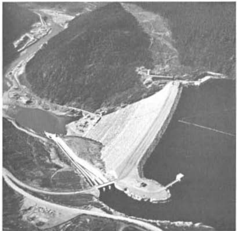
MICA PROJECT, an aerial view of all facilities, September 1976.
