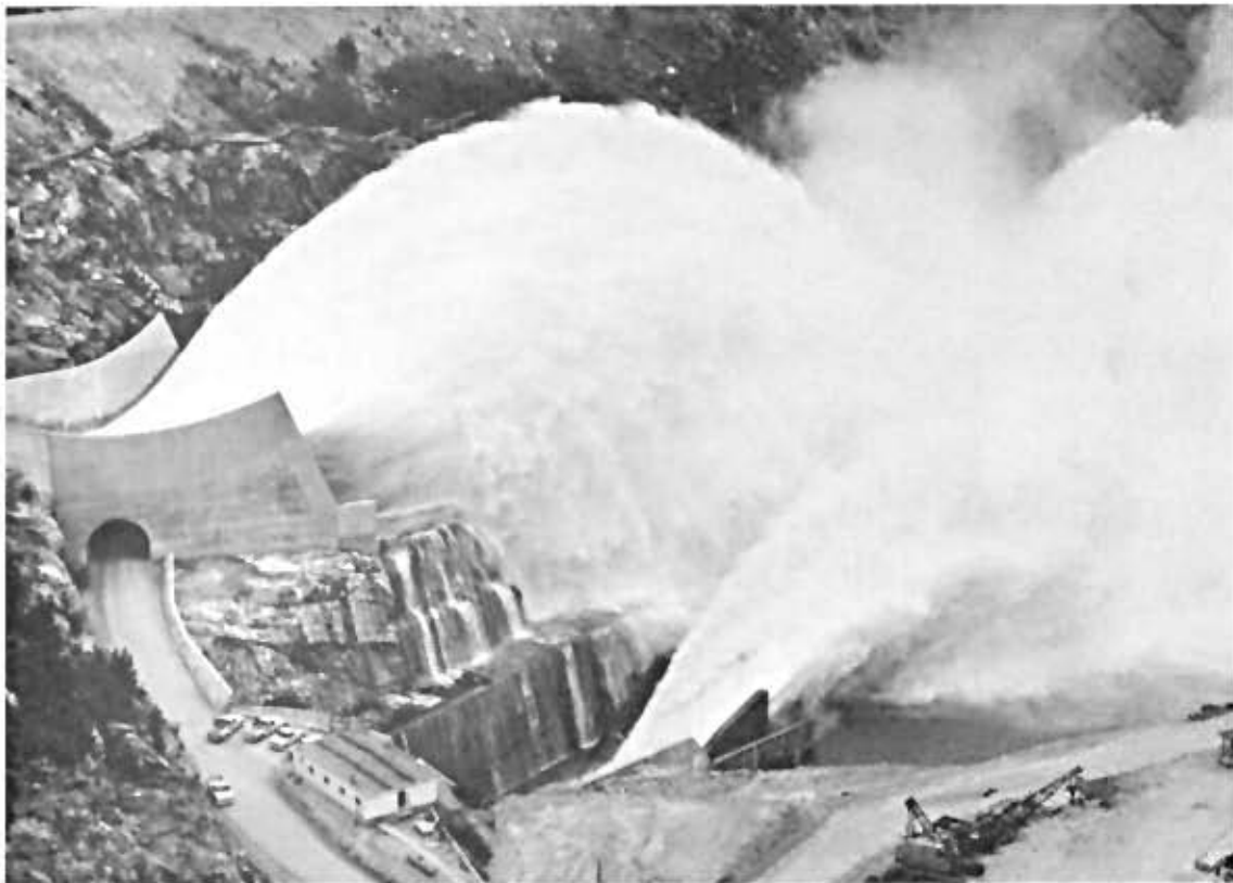
CHUTE SPILLWAY and outlet works in operation at Mica Dam, July 1976.
