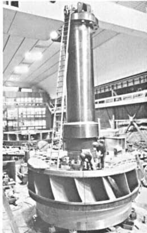
TURBINE RUNNER ready to install in Mica powerhouse.
