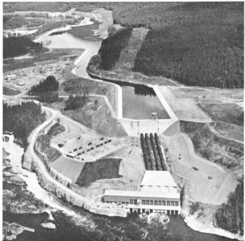
KOOTENAY CANAL PLANT in British Columbia benefits from storage at Libby and Duncan projects.
