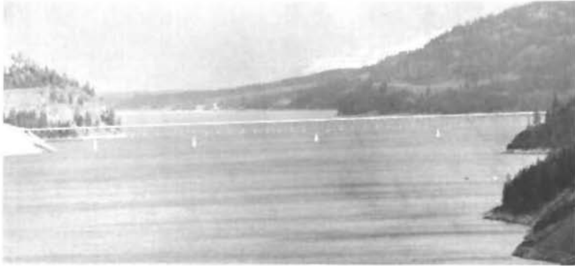
RESERVOIR BRIDGE across Lake Kootenai in Montana.
