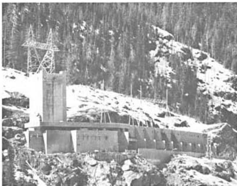
SWITCHGEAR BUILDING and tourist facility at Mica project.
