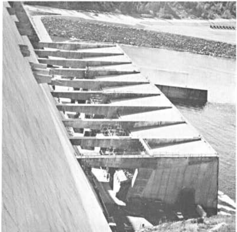
POWERHOUSE at Libby Dam.
