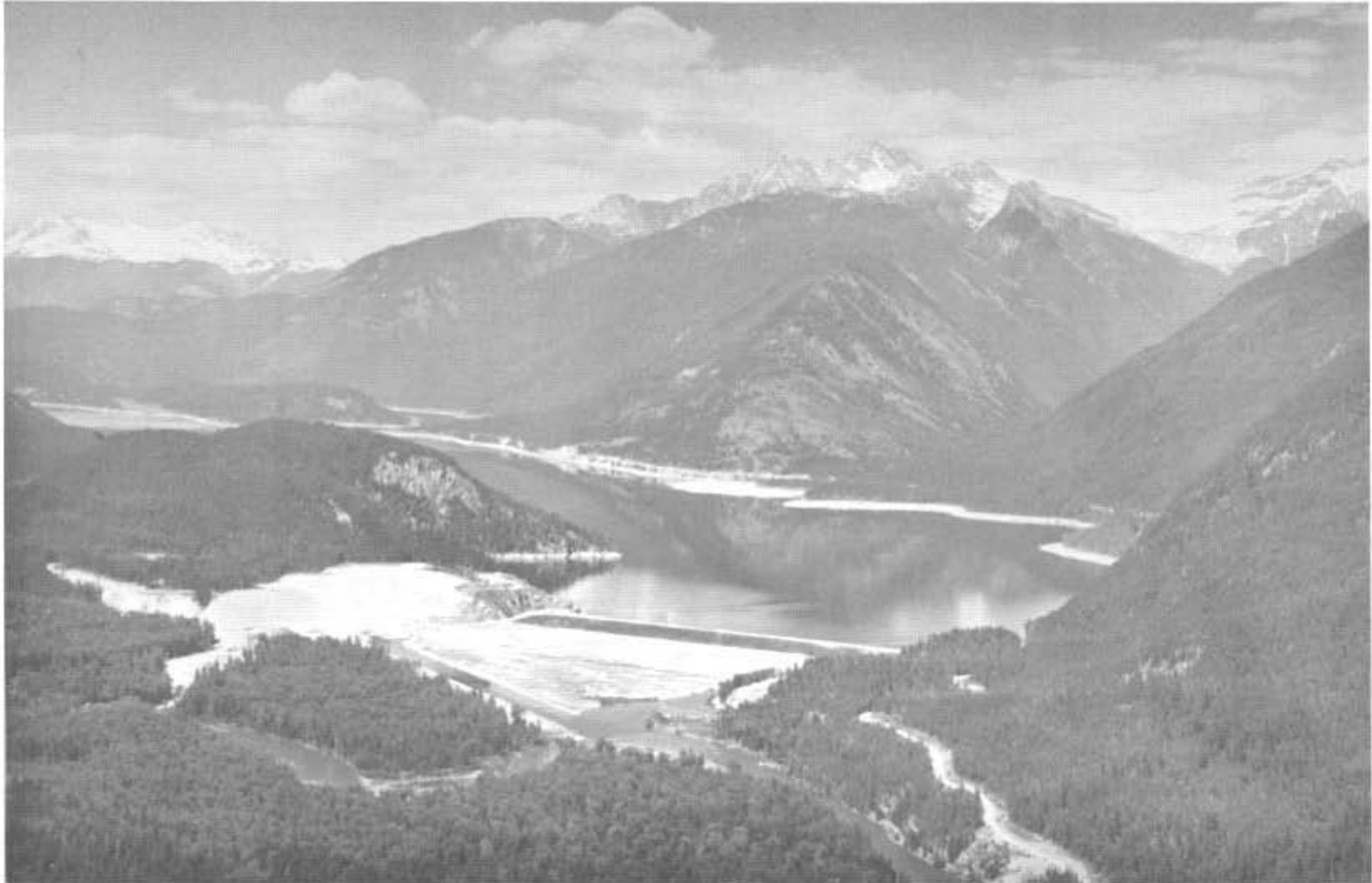
DUNCAN DAM Tunnels in the rock to the left of the dam discharge water from Duncan Lake.
