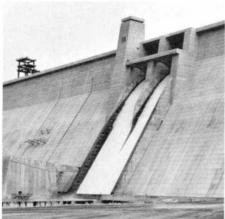
LIBBY DAM SPILLWAY and Treaty Tower,
