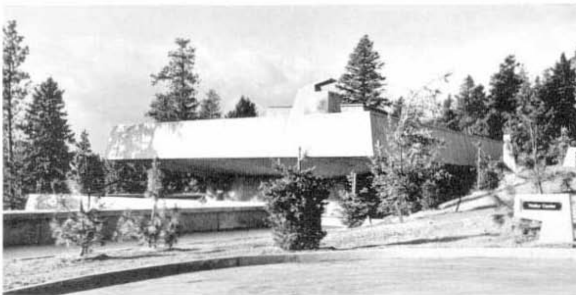
VISITOR CENTRE at Libby Dam, opened.
