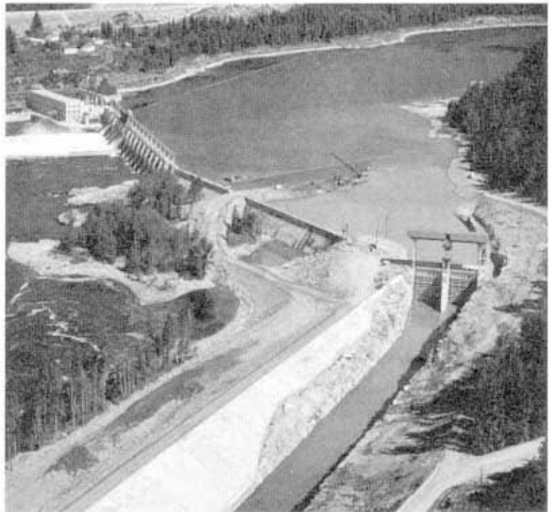
CORRA LINN DAM and forebay with canal for Kootenay Canal project.
