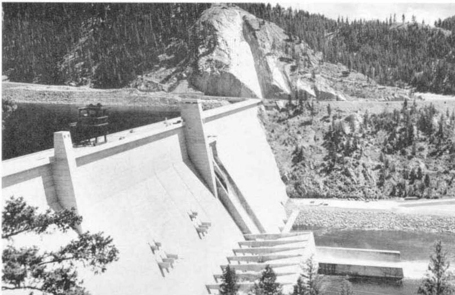
LIBBY DAM The dam and powerhouse.
