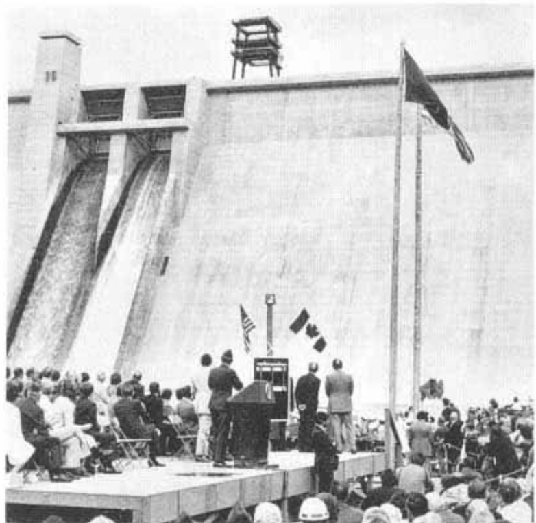
LIBBY DAM DEDICATION Spilling stops as water is diverted to generators. 24 August 1975.
