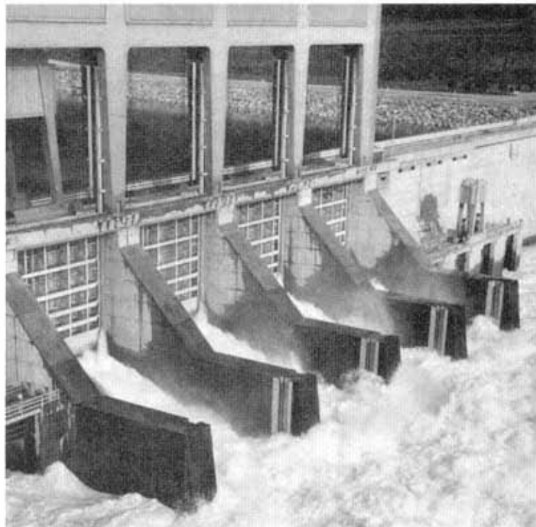
SLUICEWAYS operating at Hugh Keenleyside Dam.
