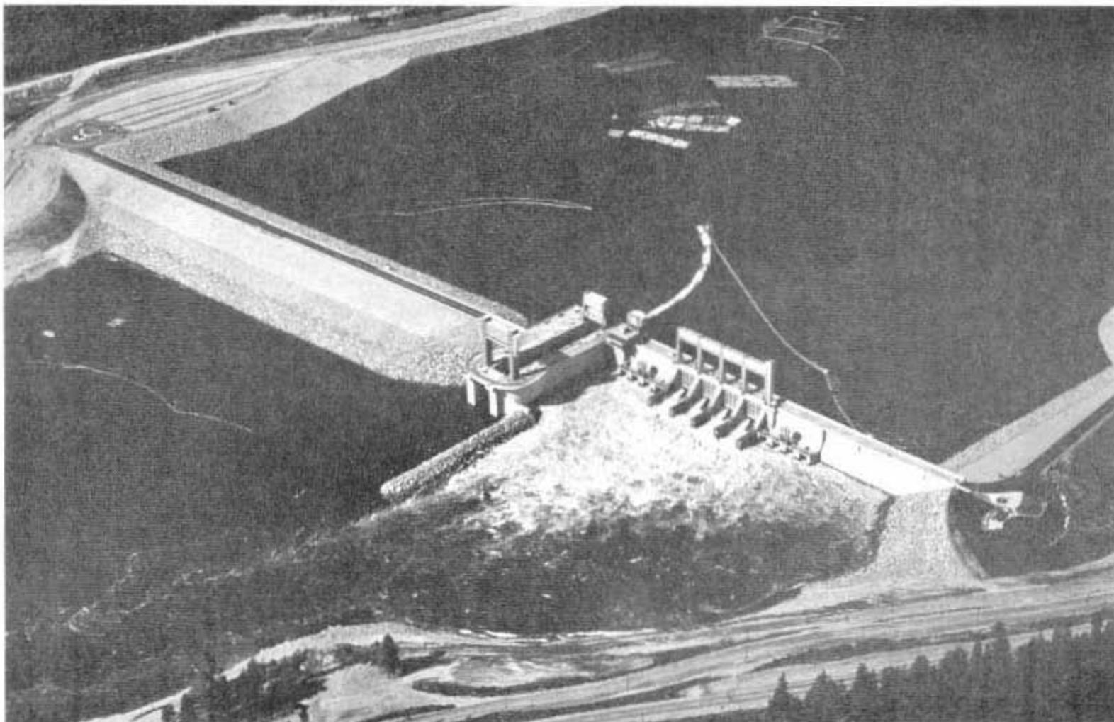
HUGH KEENLEYSIDE DAM
