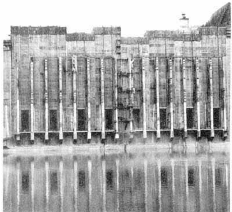
SELECTIVE WITHDRAWAL structure at Libby Dam. Construction commenced before initial filling.
