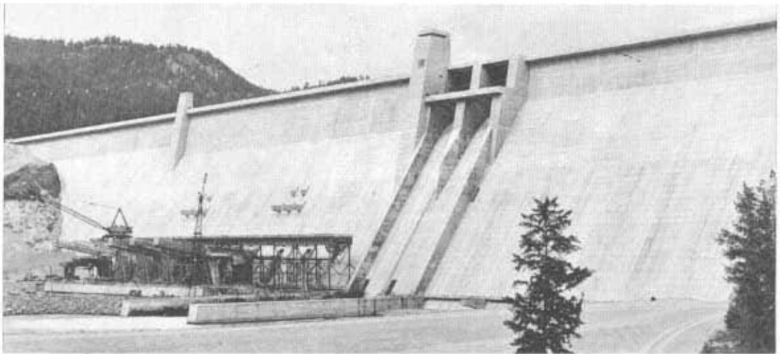
LIBBY DAM and powerhouse.
