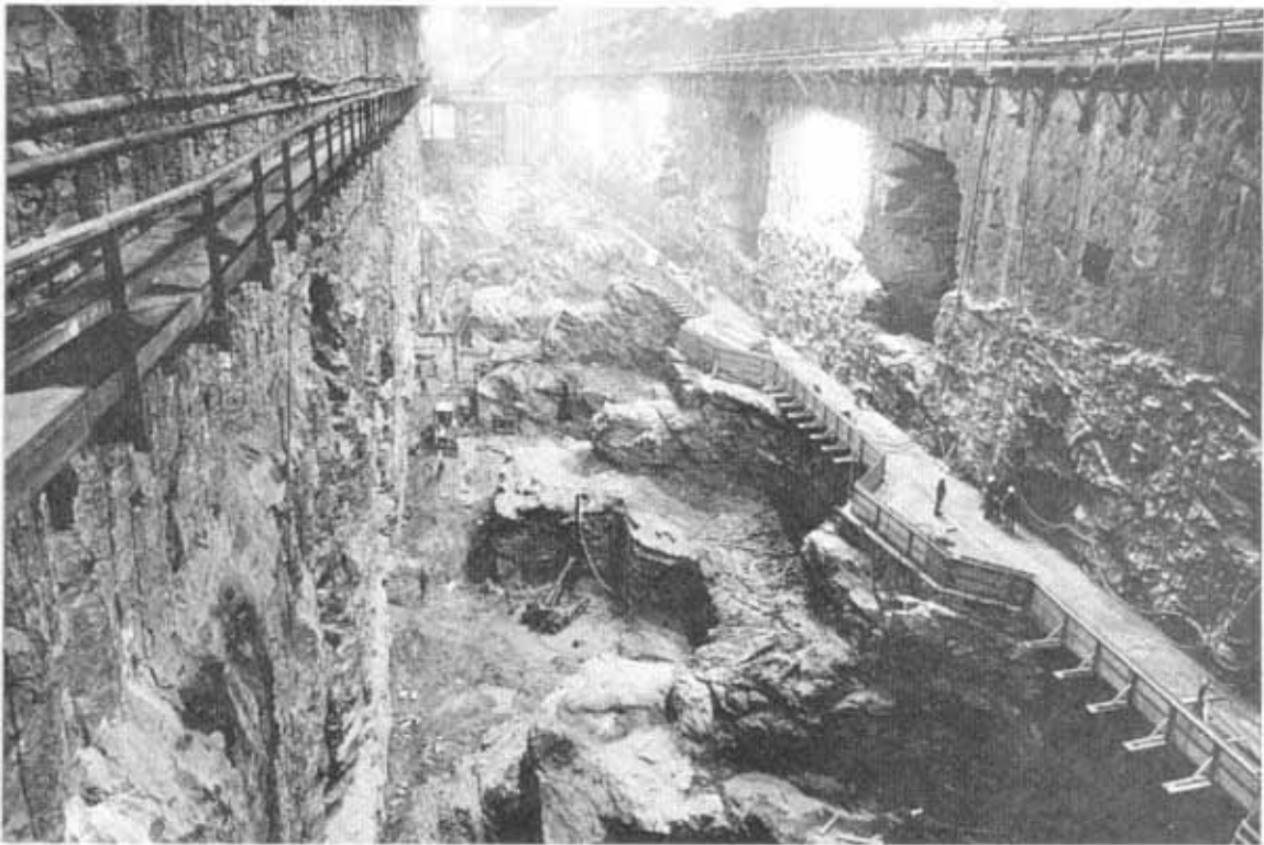
MICA POWERHOUSE underground machine hall being excavated in the rock of the west abutment. July 1974.
