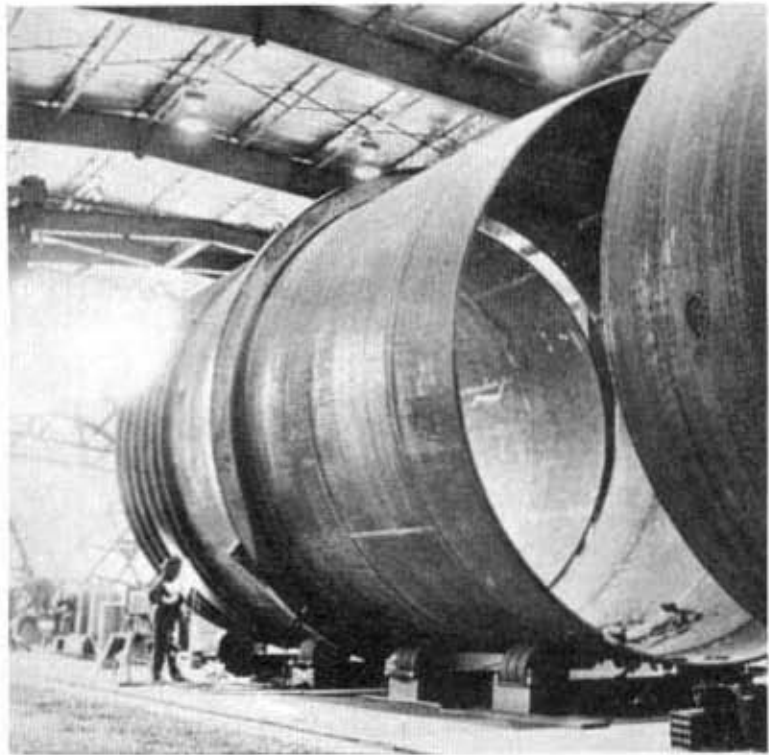
MICA PENSTOCKS, liners being assembled at site. June 1974.
