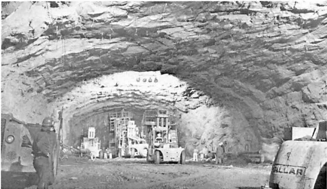
MICA POWERHOUSE excavation.
