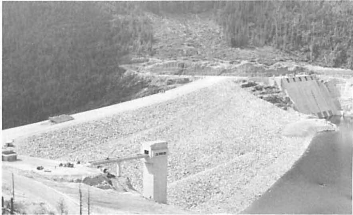
MICA DAM upstream face, outlet works tower and power intakes.
