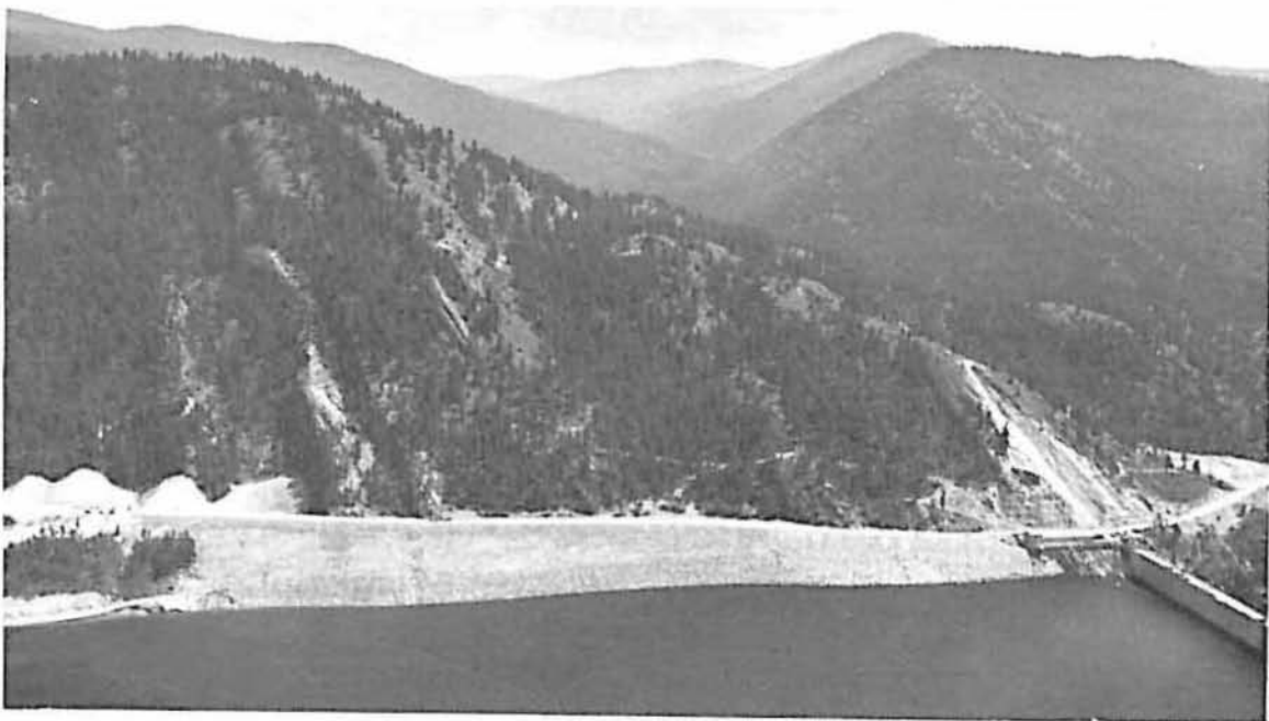
LAKE KOOCANUSA and left abutment of Libby Dam showing relocated highway and potential slide area. July 1972.
