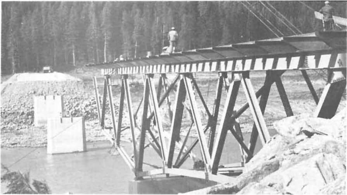
MICA ACCESS BRIDGE crossing Columbia River, part of road to powerhouse. September 1972.
