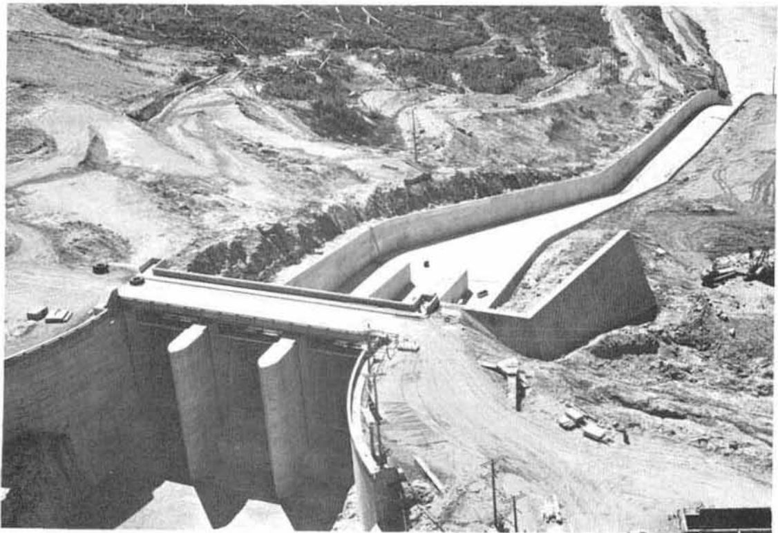
MICA SPILLWAY control structure and chute.
