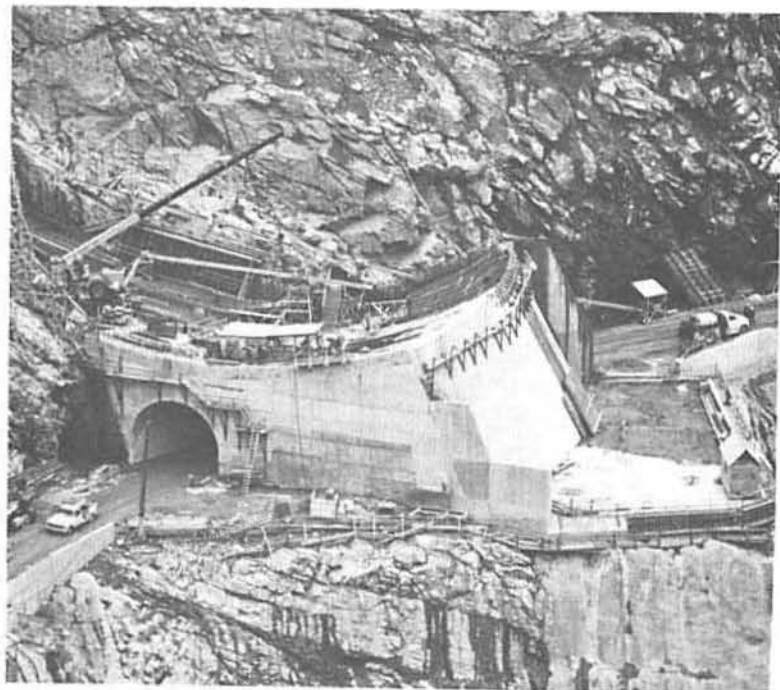
MICA SPILLWAY flip bucket nearing completion. June 1972.
