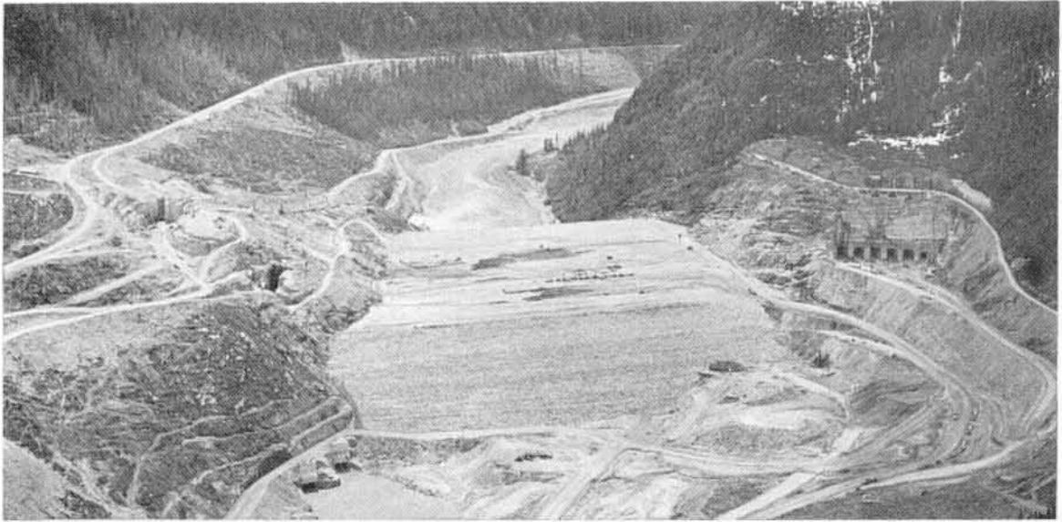
MICA PROJECT Viewed from upstream showing dam, power intakes and spillway control works. May 1971.
