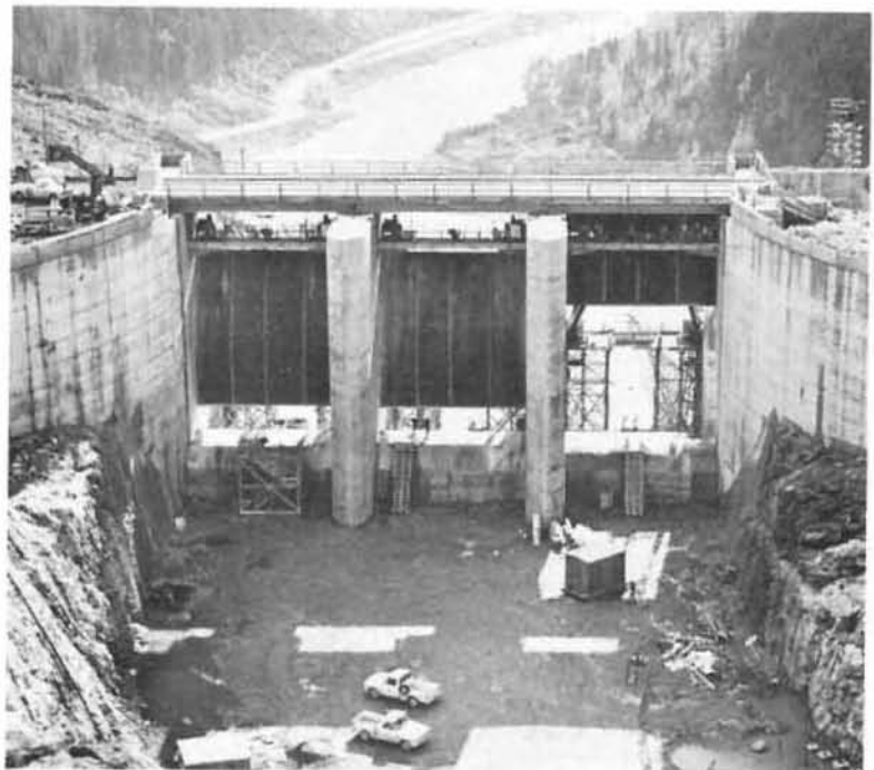
MICA PROJECT Spillway control structure from upstream. October 1971.
