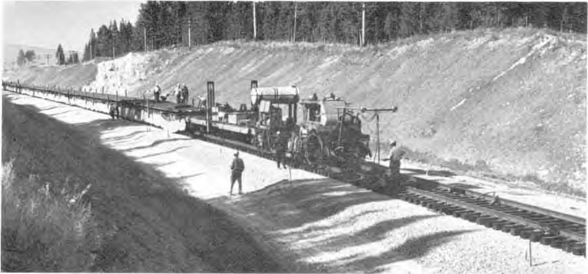
RAILWAY RELOCATION – Libby Project. Head of train carrying rails welded into lengths one-quarter mile long. August 1970.
