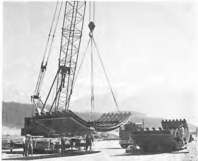
MICA PROJECT Spillway gate sections, July 1970.
