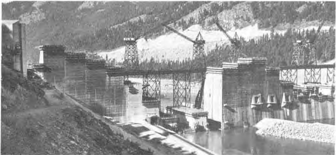
LIBBY PROJECT Upstream face of dam at left bank with diversion through monolith 33, railroad tunnel and ports for low level outlets. August 1970.
