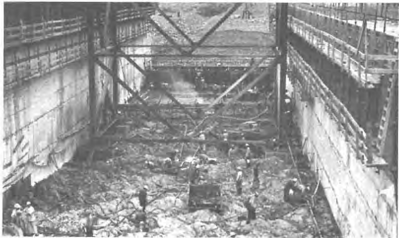
BEDROCK PREPARATION at the Libby Project. Footings for monolith 32 being prepared for concrete placement. September 1968.
