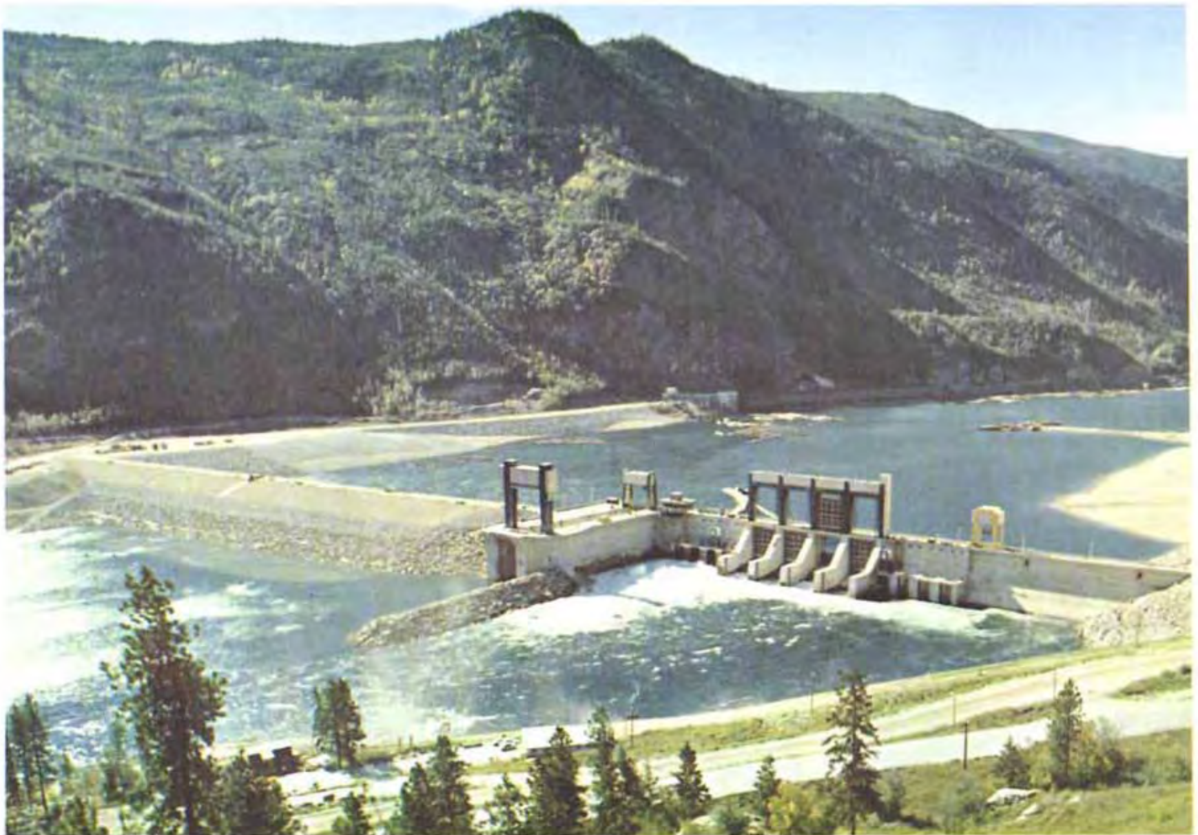
ARROW DAM — the second of the Treaty projects to be completed.
