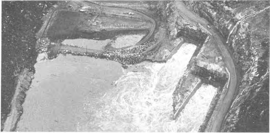
DIVERSION TUNNELS — Discharging the 1968 freshet past the site of Mica dam. June 1968.
