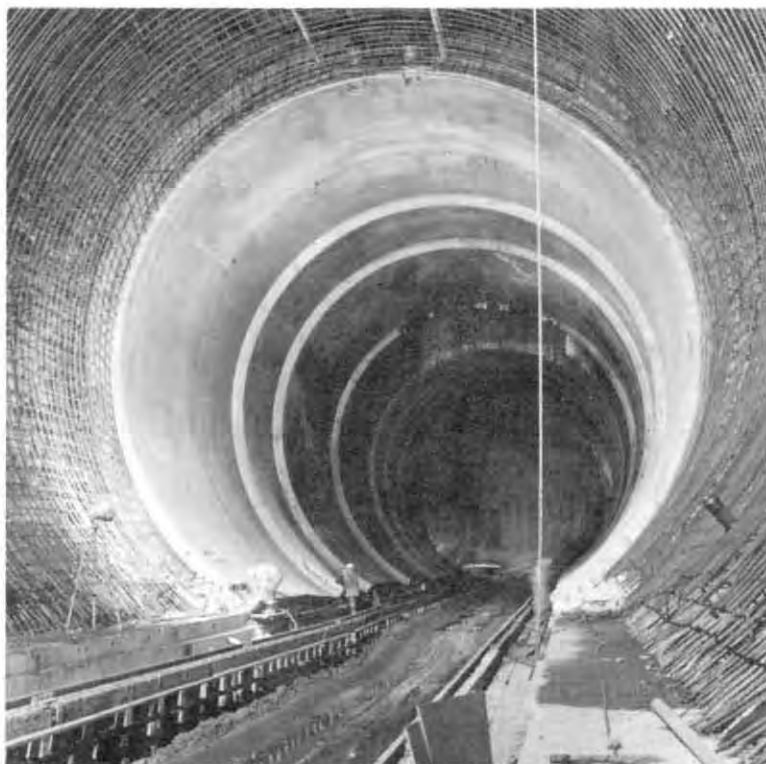
DIVERSION TUNNEL No.2 at the Mica Project. Looking upstream at the serrations for one of the tunnel plugs. 24 May 1967
