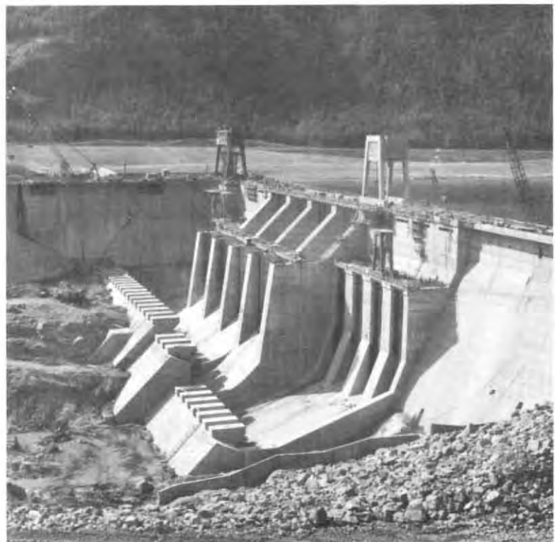
DISCHARGE WORKS at the Arrow Project. The downstream faces of the spillway openings, the low- level ports, and the energy dissipators. 6 September 1967
